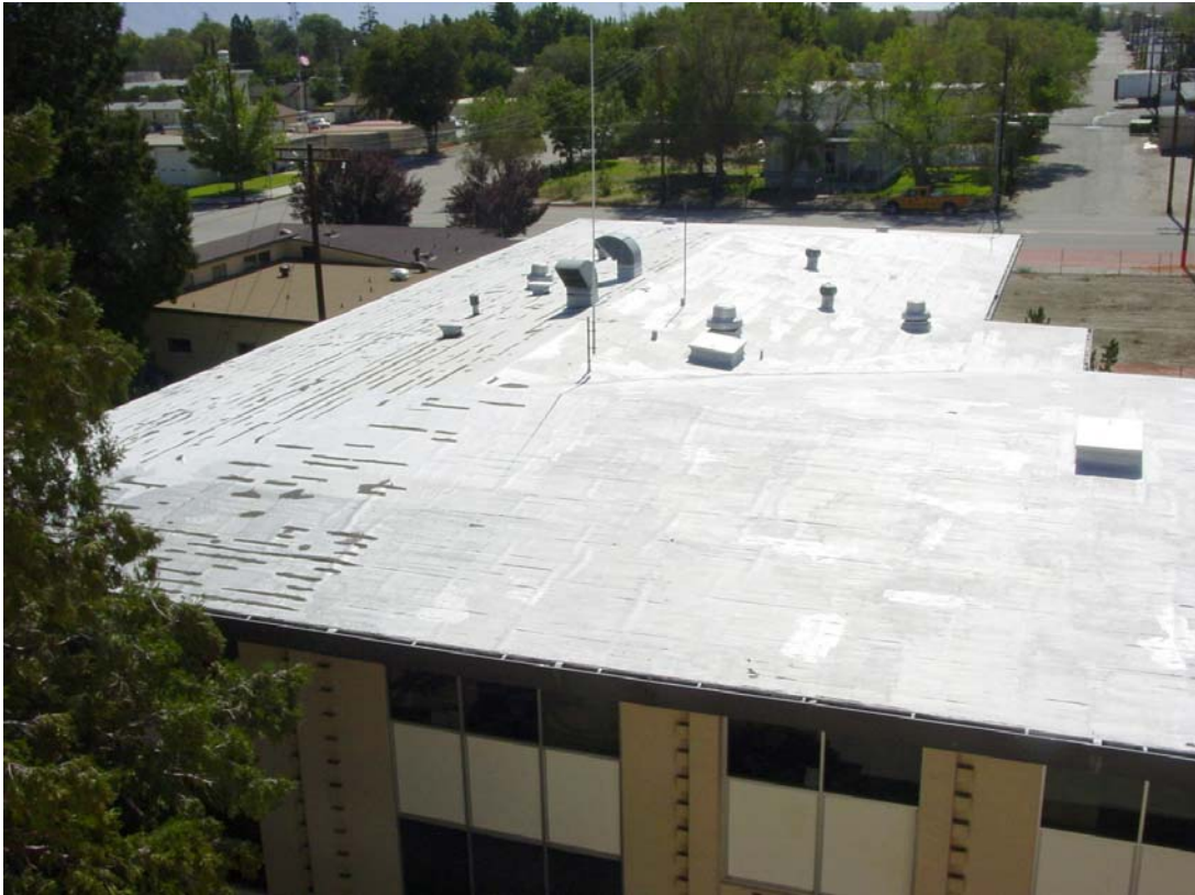
Courthouse Annex Roof, 168 N. Edwards St. Independence, CA
