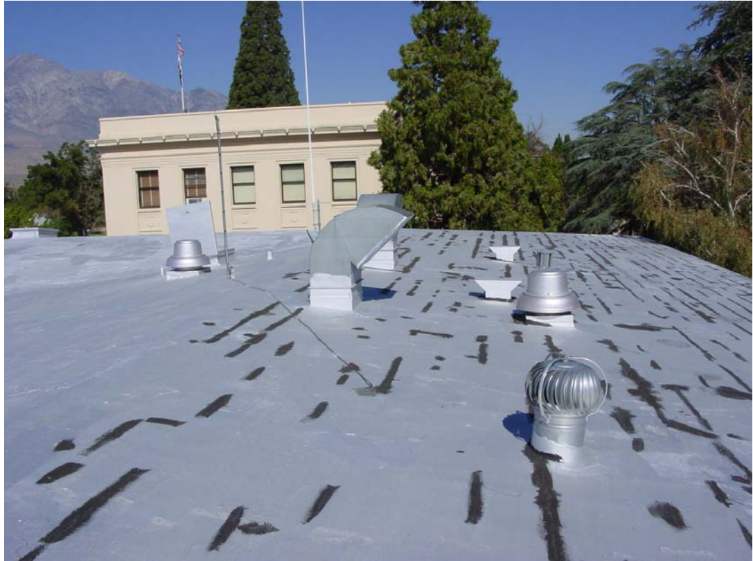
Inyo County Courthouse Complex Re-roofing Project Photographs Page 1
